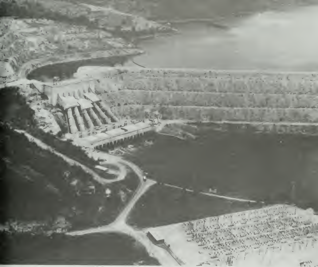
Hydroelectric sluices in the Akosombo Dam Courtesy Embassy of Ghana, Washington
